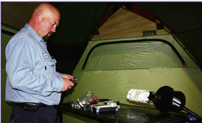
Substation Technician Jason Olinger splices fiber to restore Internet, telephone and cable television services to customers during a storm.
